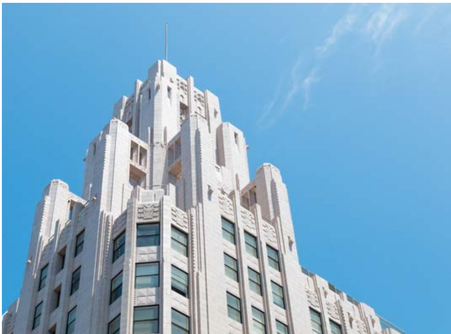
The Title Guarantee & Trust Building in Los Angeles. Architectes : John et Donald Parkinson.
